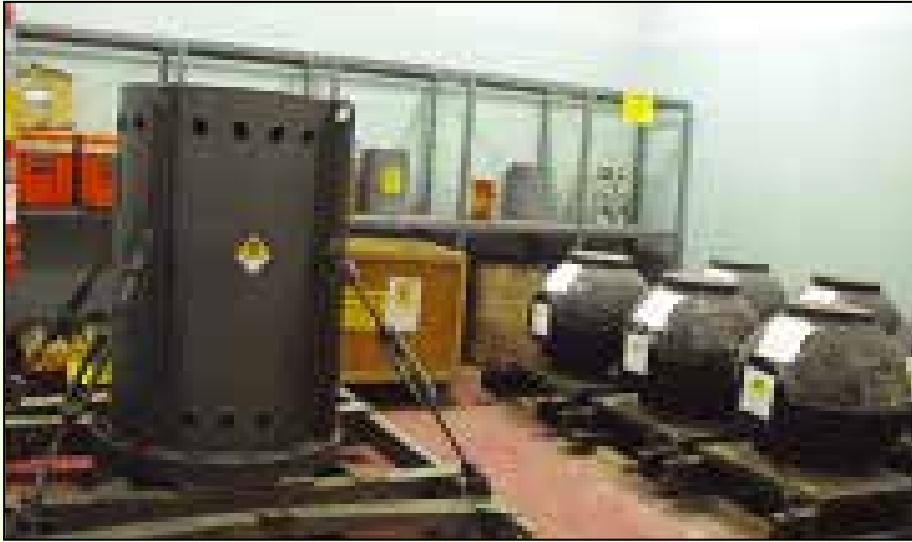
Storage of Disused Sealed Radioactive Source at CWPSF
